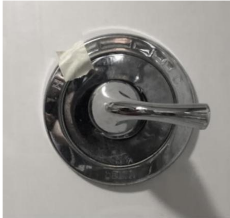
Figure 14. The single-handle pressure balance valve knob set in “off” position.
