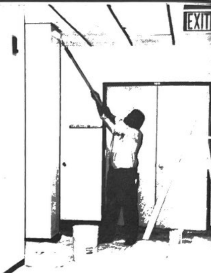
Campus crews were busy during the semester break sprucing up the place, painting campus buildings and enhancing the overall look of CCSU. John Saldivar, painter, was caught in the act in Center for the Sciences applying a fresh coat of paint. Other additions include landscaping at the University's entrance sign.
