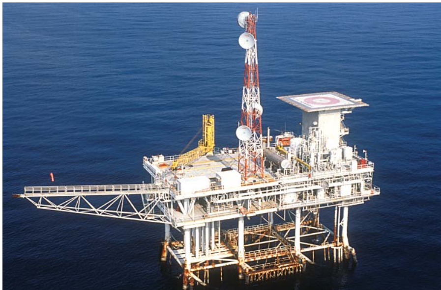
Figure 1. Mobil’s High Island A389 platform.
